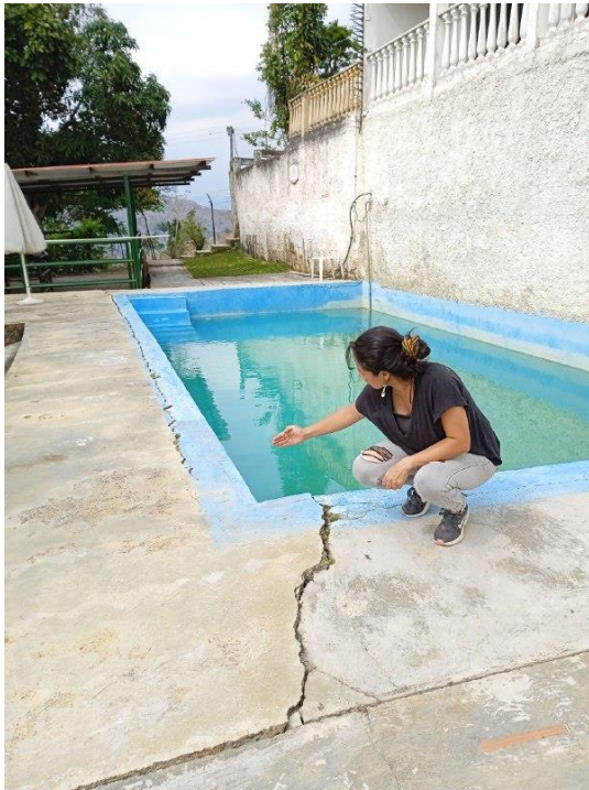
Due to deterioration, cracks in the cement, the pool was closed for a period of time.
